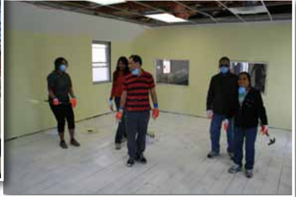
Painting newly-installed drywall
