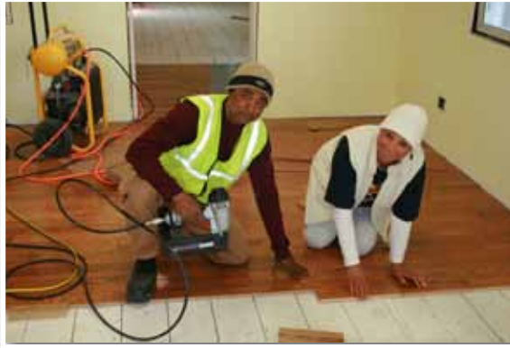
Installing new flooring
