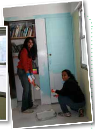
Repainting walls and woodwork
